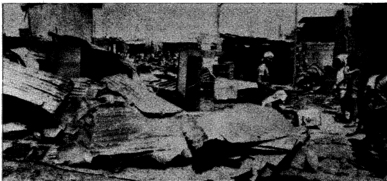
Cutted remains of Tondo. The tragedy has been traced to a rash of "urban renewal" fires linked to the Zonal Improvement Program scheme. (AK Photo)
