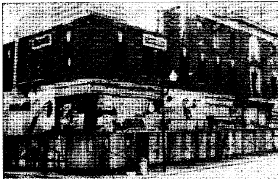
What's left of the structure — an empty shell. Soon demolition will be over, leaving no trace of the building. But the memory of the tenants' struggle to keep their hotel will live on, etched in people's history. (S.F. Journal)
