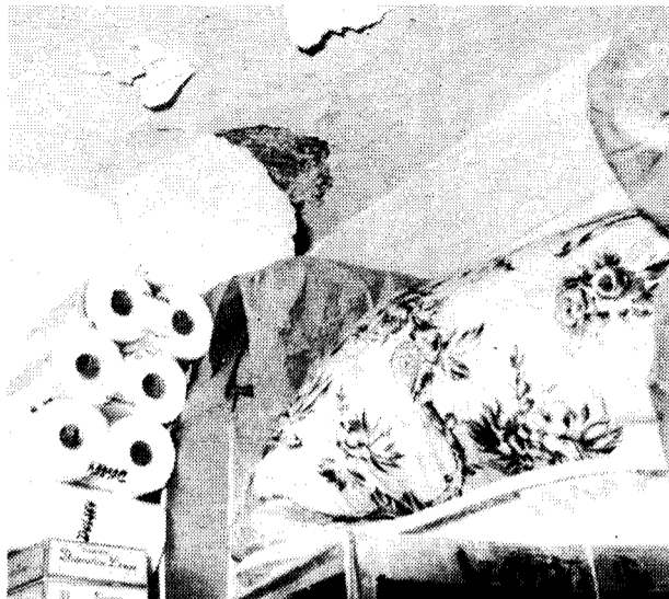
Some of the numerous health and safety violations in the Milwaukee Hotel which were ignored by the owners. With the tenants' management of the Hotel these violations would be corrected. [AK photos]
