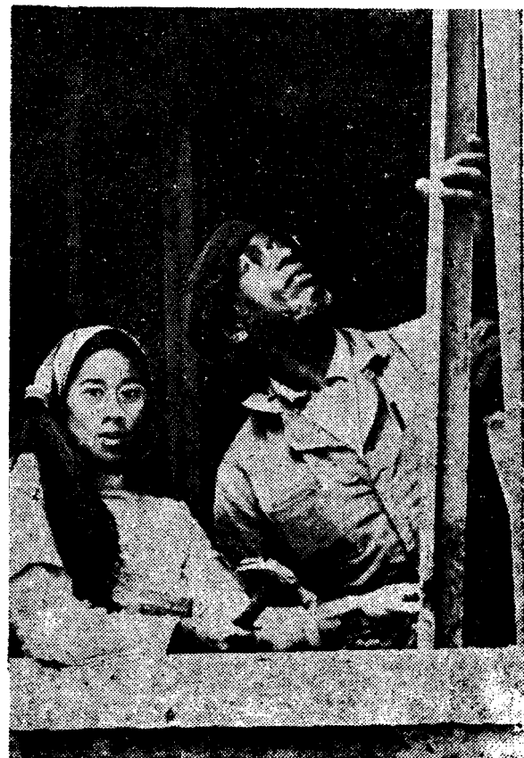
Contractor works on window with Cleanup crew
