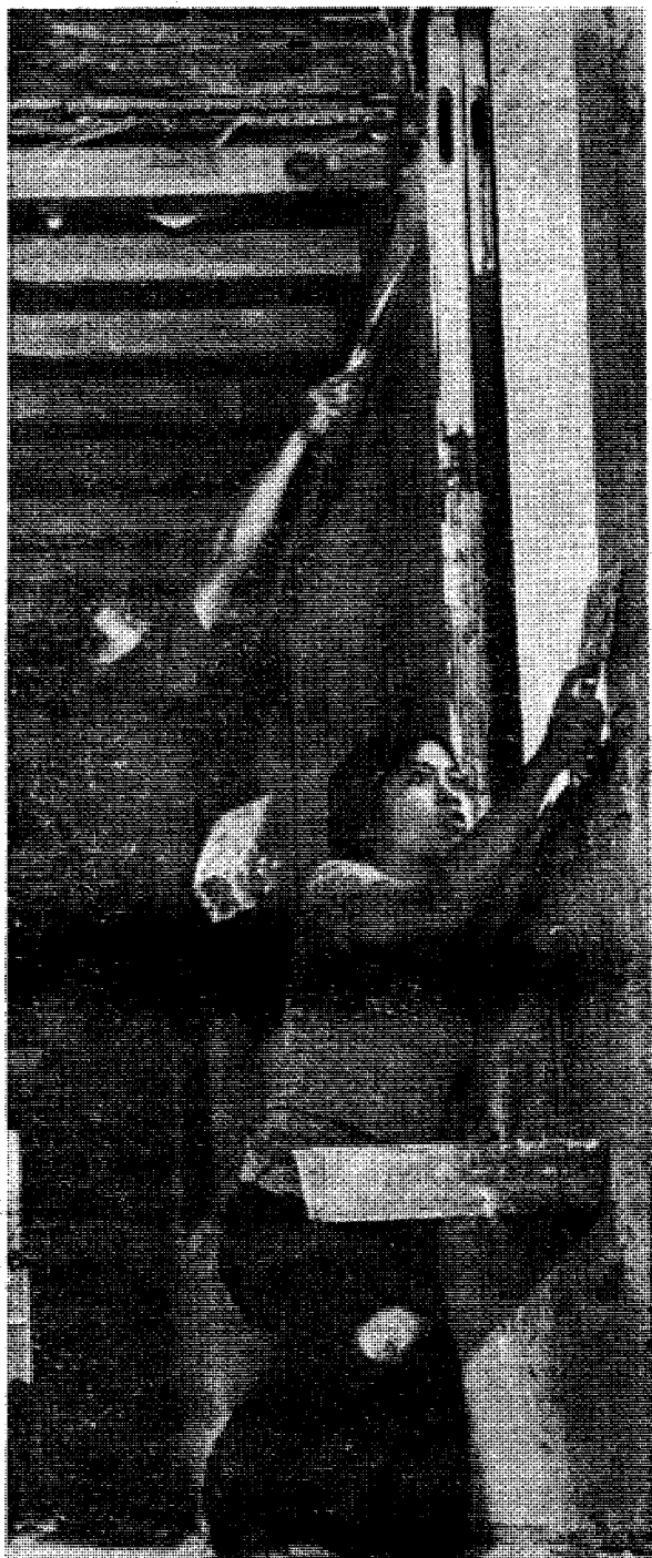
Youth Council members refurbish hotel corridor
