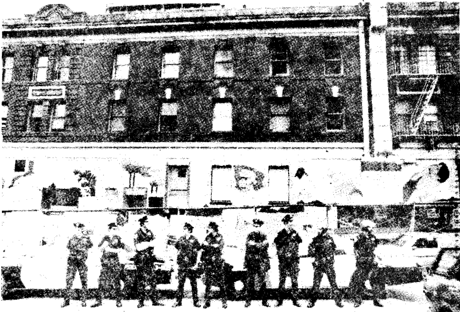
Since its tenants violent eviction by the S.F. Police, the I-Hotel has been heavily guarded. Despite the city's order to halt demolition pending decision on the validity of the demolition, the Grange Debrise Co. still proceeded to smash the hotel's back wall. [S.F. Journal photo]
